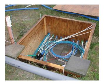
Figure 6. End of the IEC trajectory with Y-connector and termination box
