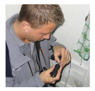
Figure 19. Pushing ferrule holder into connector housing
