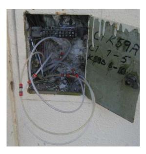
Figure 15. Existing wall boxes with extended microducts, hanging out temporarily
