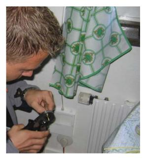
Figure 18. Crimping cylinder around ferrule holder
